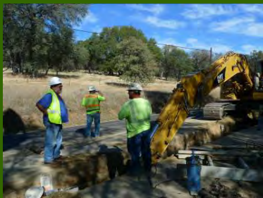
Revitalizing the wastewater collection system
