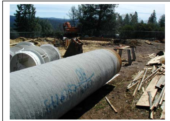
Pleasant Oak Main Replacement ($22 million)
