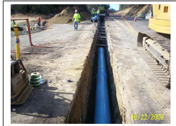
Mother Lode Forcemain Replacement ($4.5 million)
