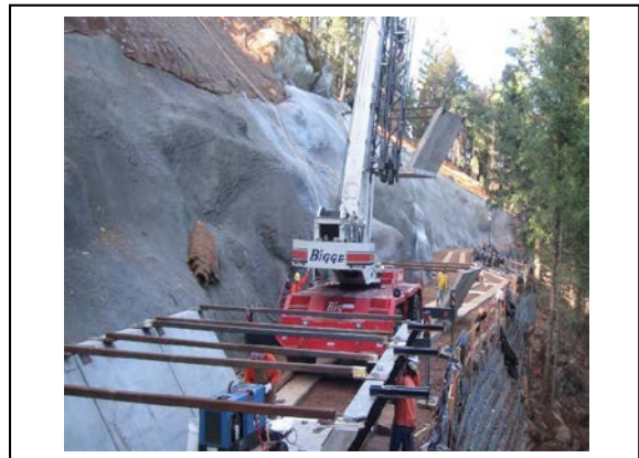
Flume 51 Replacement ($3.6 million)
