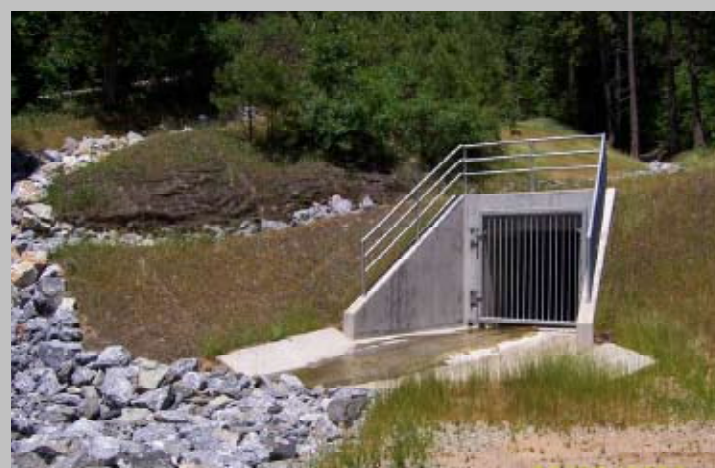
Above: Hazel Creek tunnel, renovated in 2006. Right: Wetlands that will be revegetated and expanded in 2007 as EID repairs damage and stabilizes approximately 2300 feet of channel located downstream of the tunnel. These improvements will help the District maintain the ability to transfer water from EID's hydroelectric power generation system to Jenkinson Lake in Sly Park.
