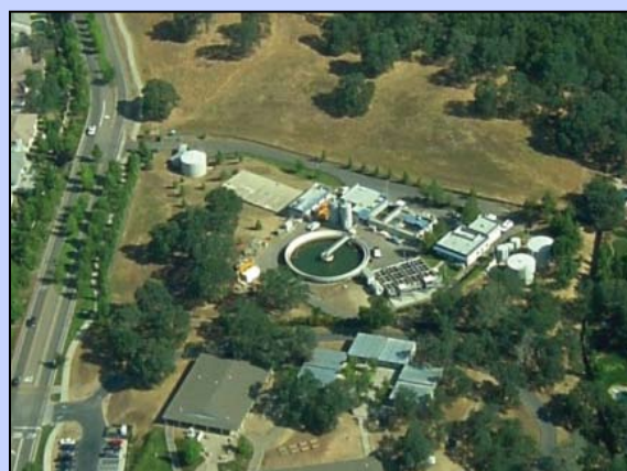
EID's El Dorado Hills water treatment plant.
