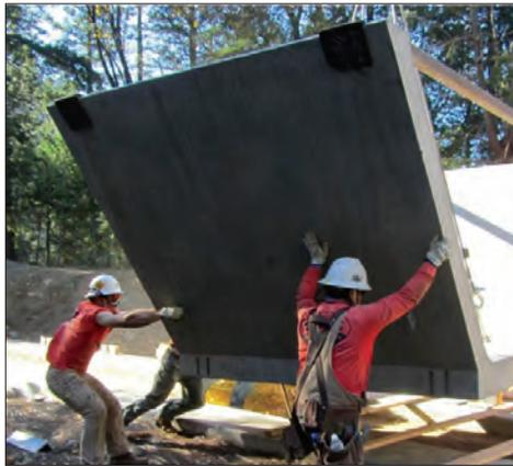
Workers place a section of pre-cast concrete flume
